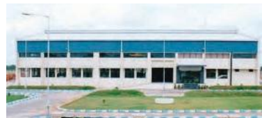
Pashamallaram Plant - Hyderabad: Power Transmission Accessories
